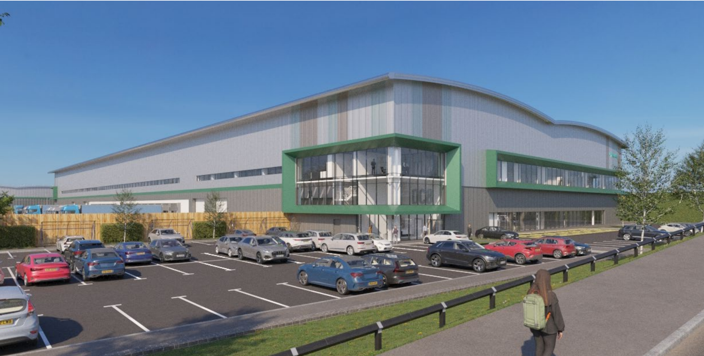
FIG 32 - DC8 (ZONE D) VISUAL - OFFICE & ENTRANCE OSBORNE ROAD
