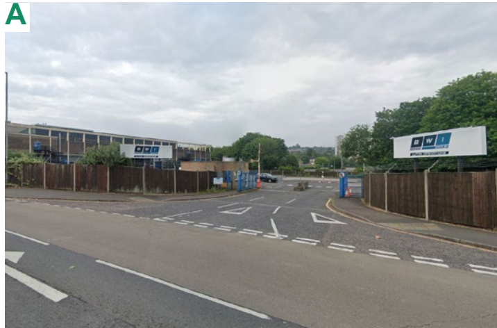
FIG 8 - EXISTING ACCESS POINT FROM WINDMILL ROAD
