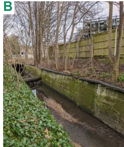
FIG 9 - RIVER LEA RETAINING WALLS
