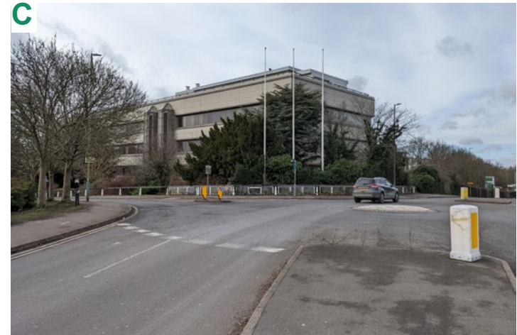
FIG 10 - VIEW FROM GIPSY LANE TOWARDS GRIFFIN HOUSE
